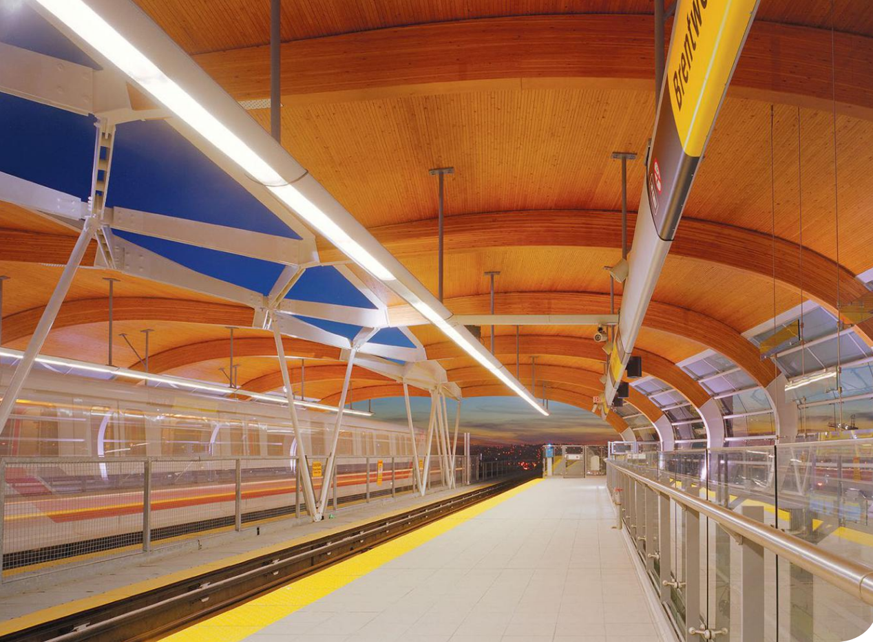
Perkins&Will used mass timber to create the roof of the Brentwood SkyTrain station in Burnaby, British Columbia. Courtesy of Perkins&Will.
