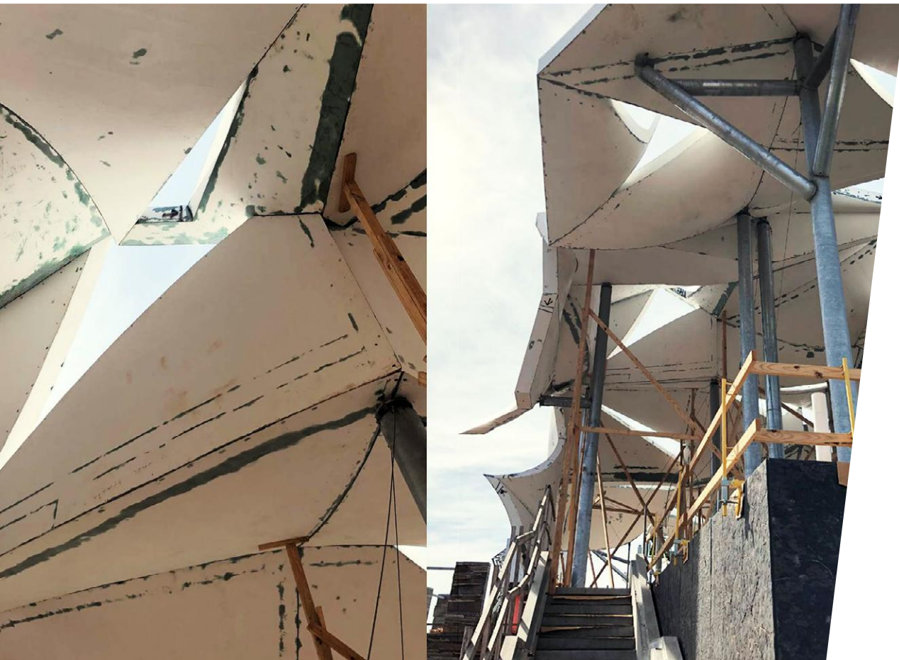
In-progress photos of the ONEOK Boathouse Pavilion in Tulsa, OK, composed of 130 sail-like, fiberglass-reinforced polymer panels. Courtesy of Kreysler & Associates.
